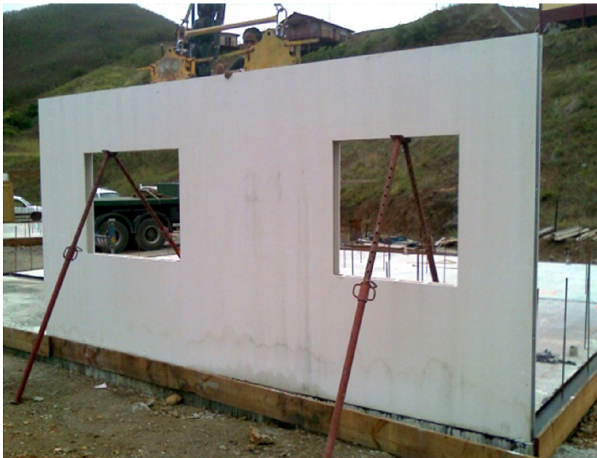
Fig. 4.6 Erection of GFRG panels over plinth beam at site
