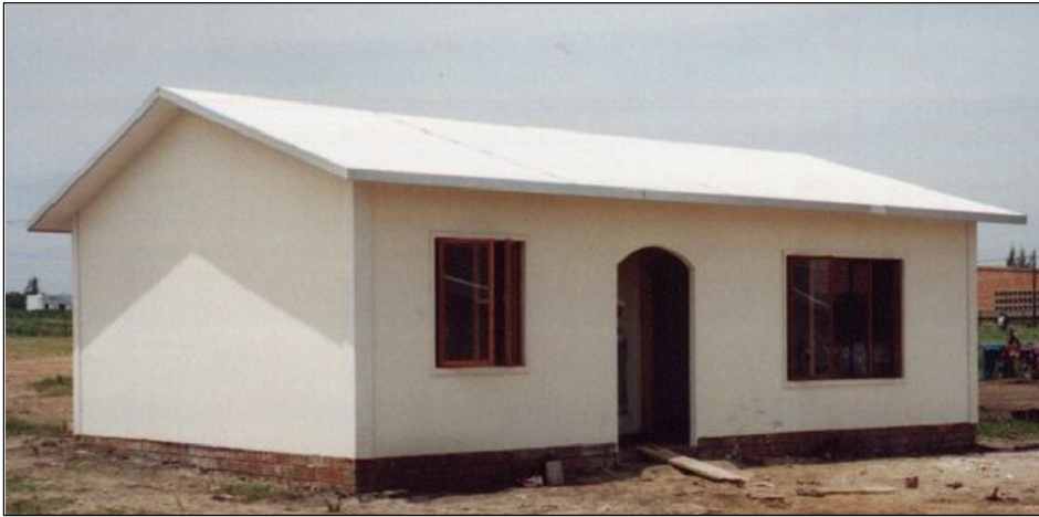
Fig. 4.5 Small GFRG house with pitched roof
